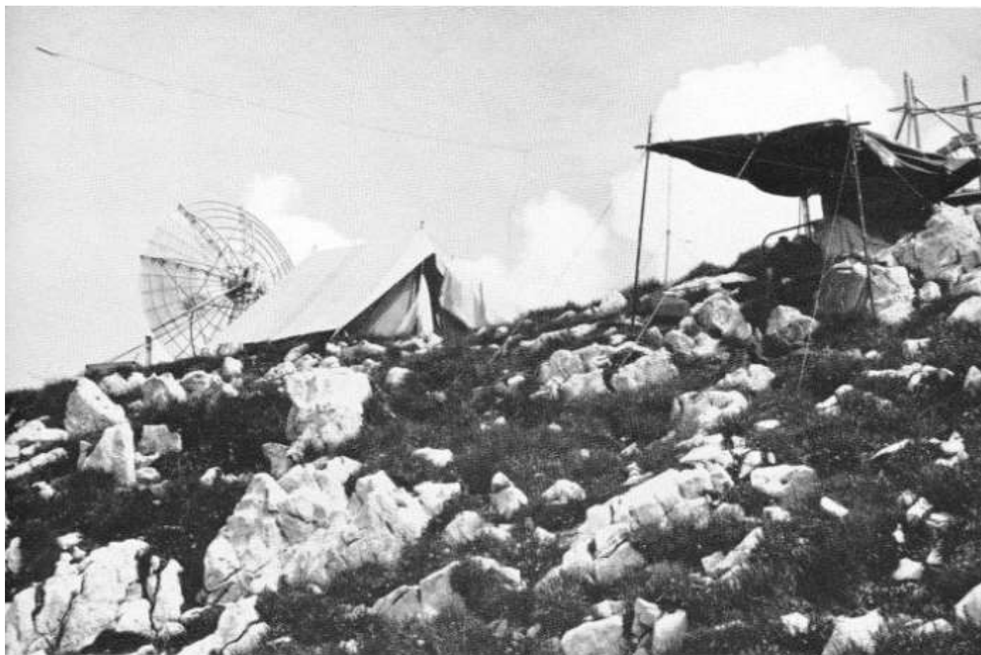
ABOVE: The station on Mt. Telegrafo, 7,277 ft., in Northern Italy. This shows the aerial, one of the tents, and the survey-style engine house on the right. There was only just room up here to make flats for the tents. The transportable 15 ft. dish aerials for both stations were made at Gateshead Works. BELOW: The one-ton jet helicopter which Heliswiss sent to make the final lifts of equipment to site on Telegrafo.
