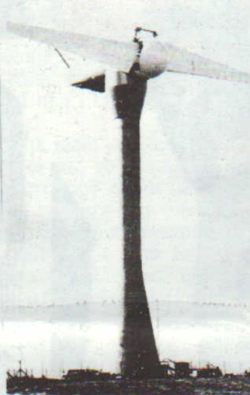
The 3 MW 60m diameter wind turbine generator.
