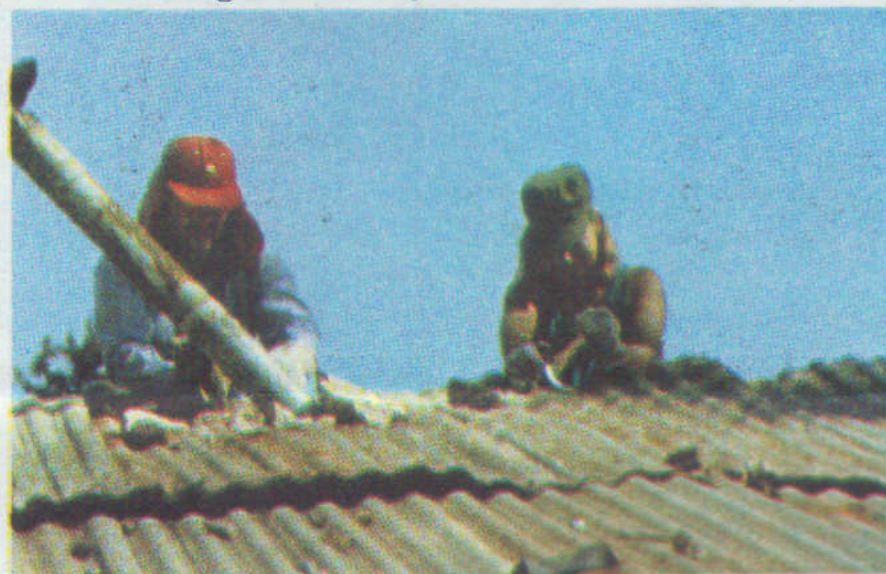
Two members of the group renovating the tuck shop roof.
