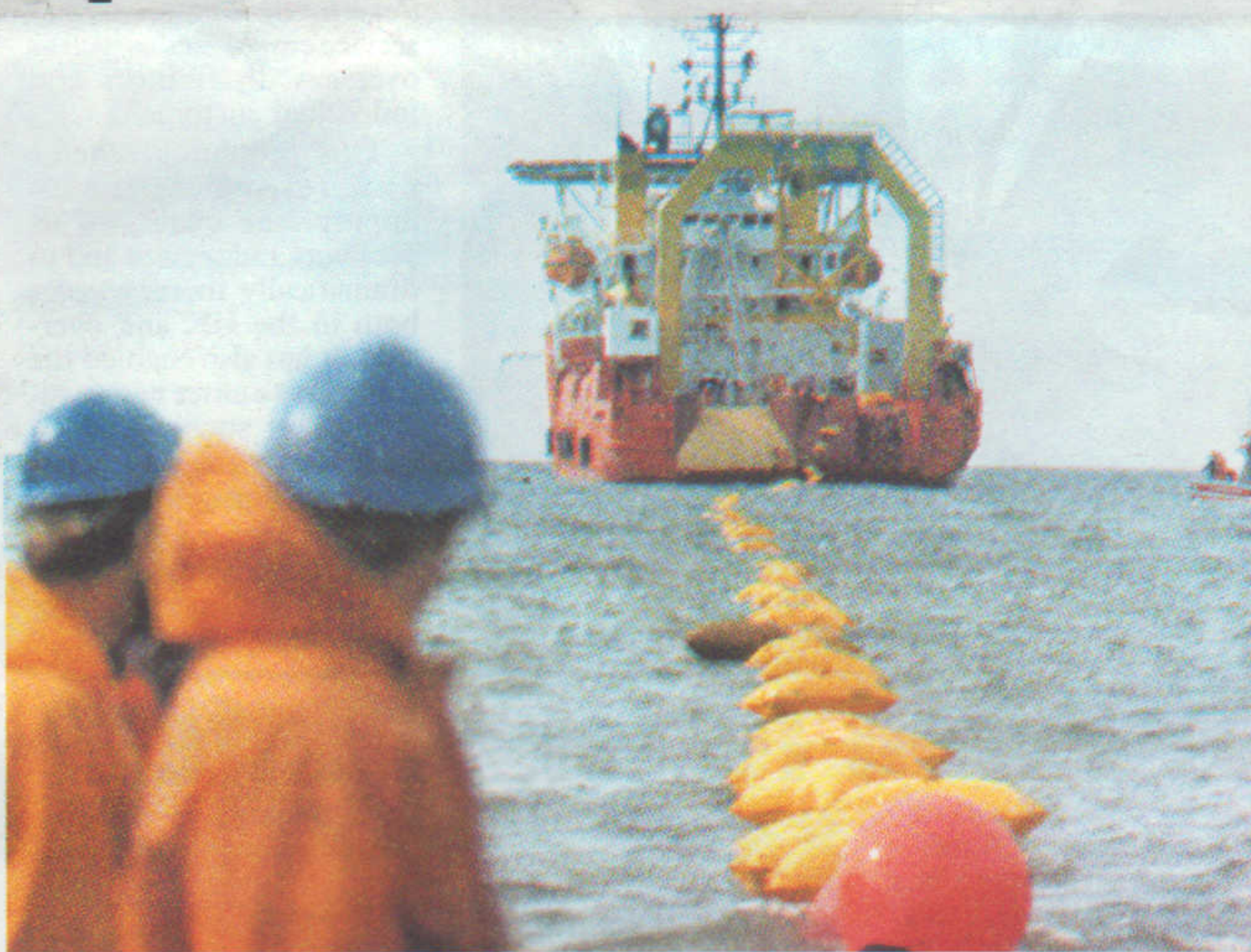
BT's Flexservice 3 ship laying the Scotland to Northern Ireland cable.
