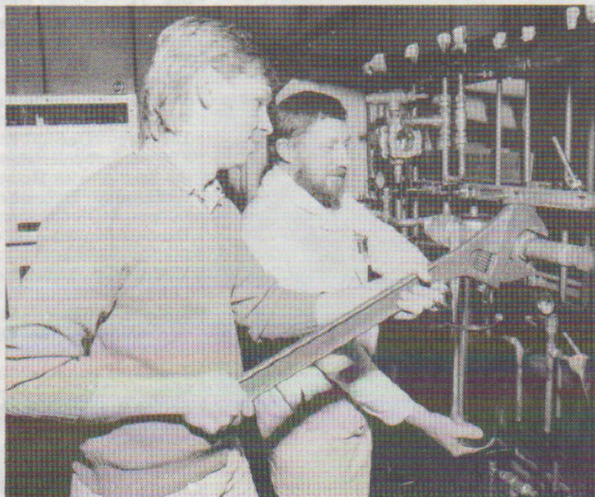
Leading hand Mick Worby and Duncan Haley use one of the Shop's giant knick-knacks to assemble a water control unit.
