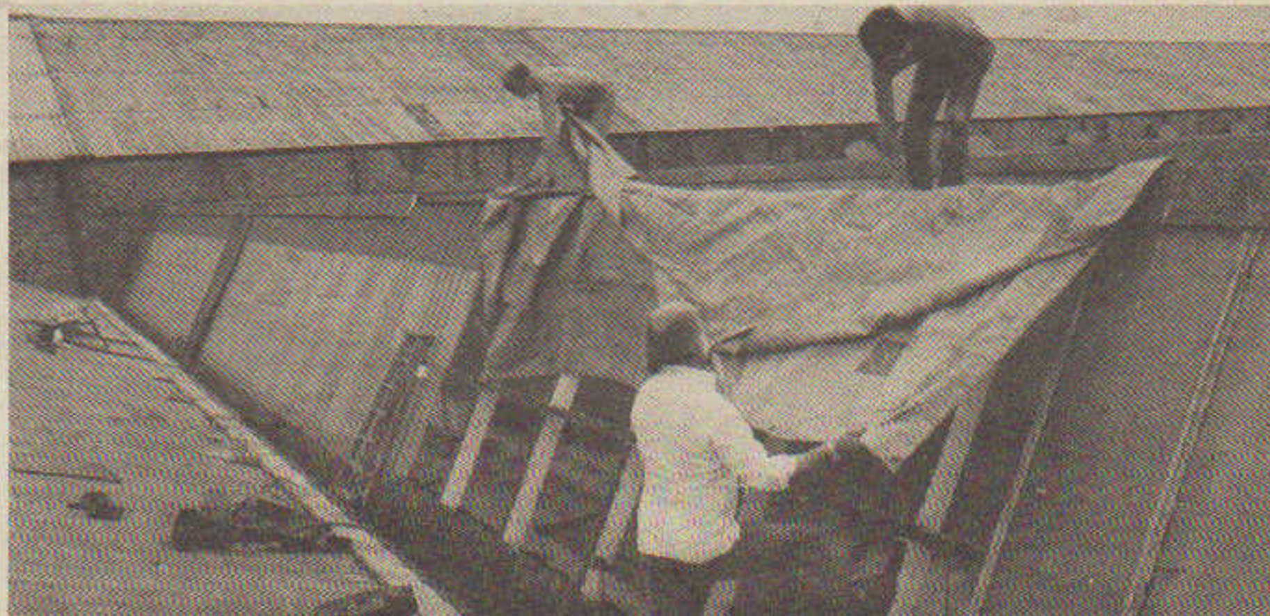
Hard at work on the roof replacement.
