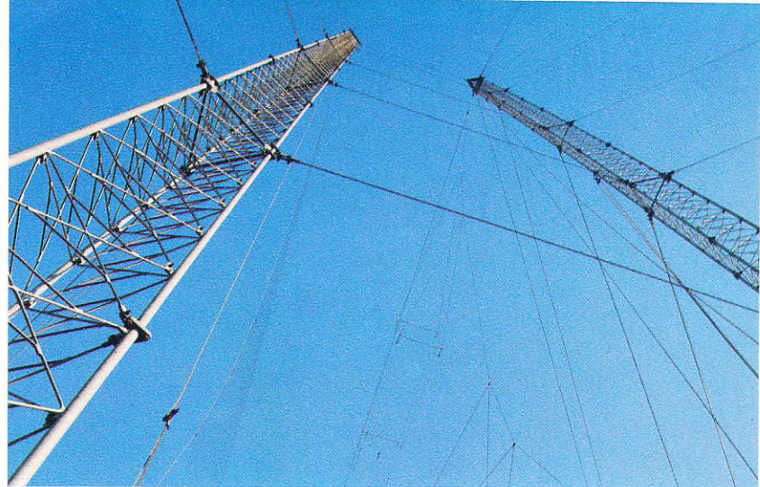
0 kW HF wideslew wideband broadcast antenna. Top left: R3010 300 kW HF switching matrix. Top right: Lightweight masts supporting R9010 antenna. Bottom left: 2 MW quarter wave MF cage monopole. Bottom right: 2 MW 6 element MF Yagi antenna.
