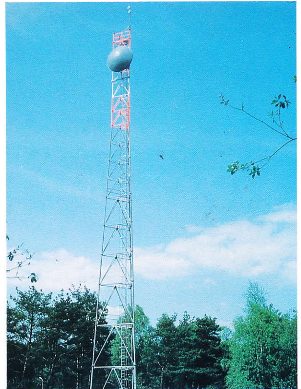
Microwave antenna support tower.
