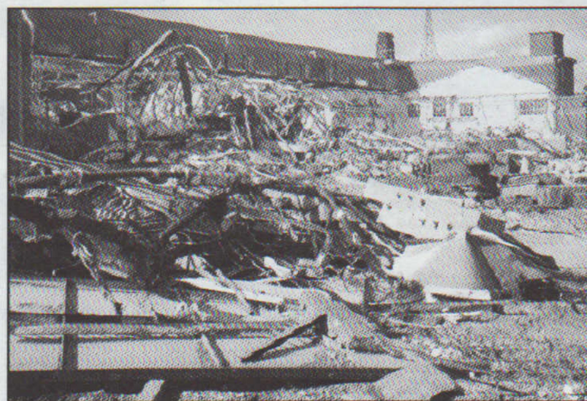
The demolition of Building 46
