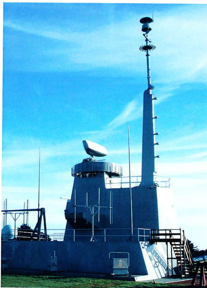
Above: the complete Pole Mast now installed at the MSETF
