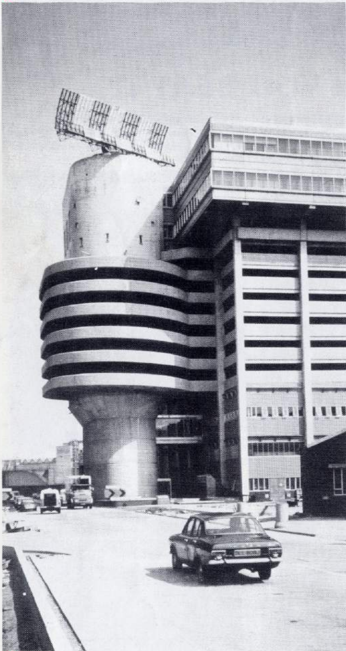
An S650, one of four MRSLS 50cm radars at London Airport. The UK airspace is covered by MRSLS radars of this type. The Company is in the process of modernising them and others throughout the world, giving them many more years of service.
