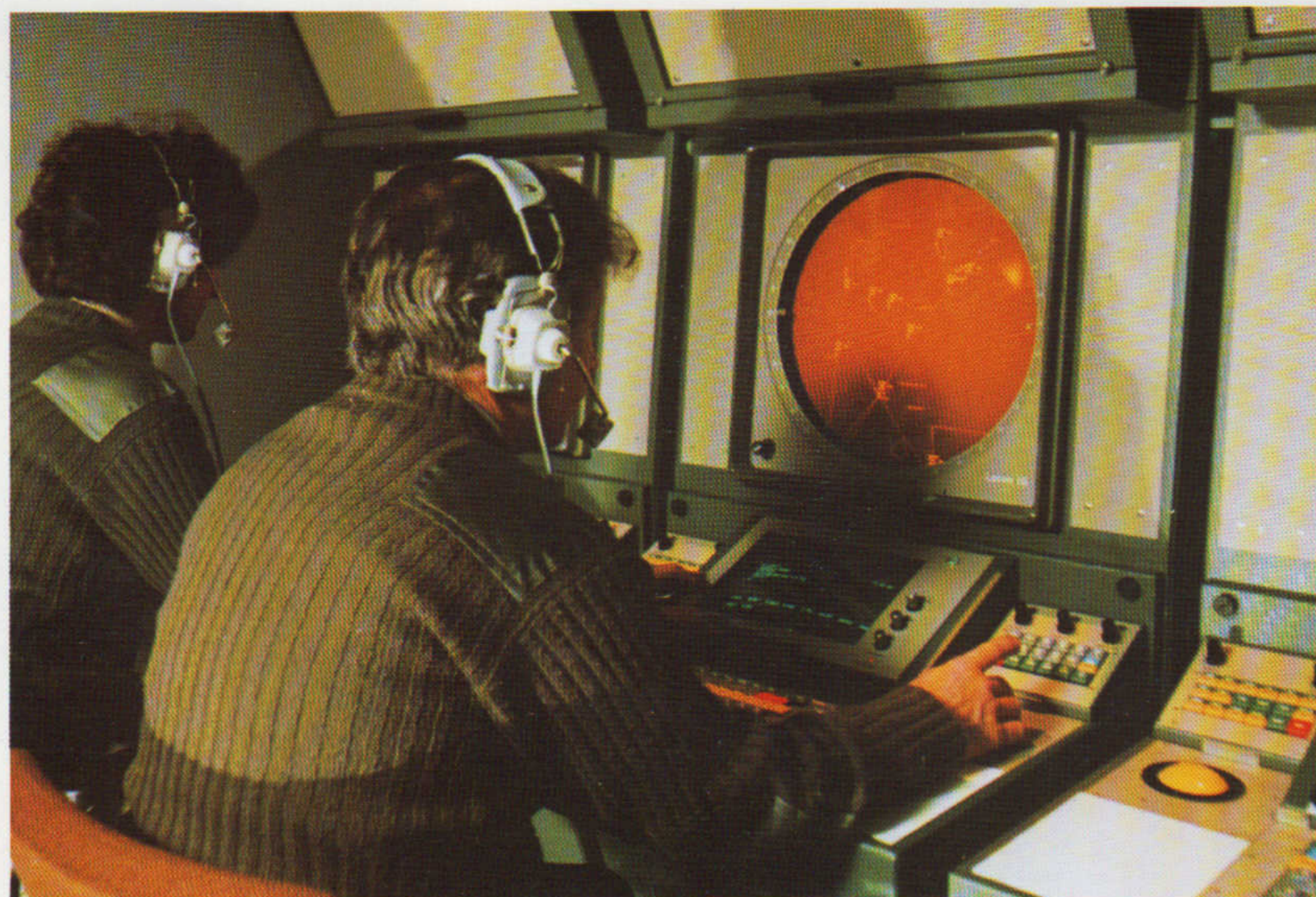
A recently exported Air Defence Display and Data Handling Cabin Installation.
