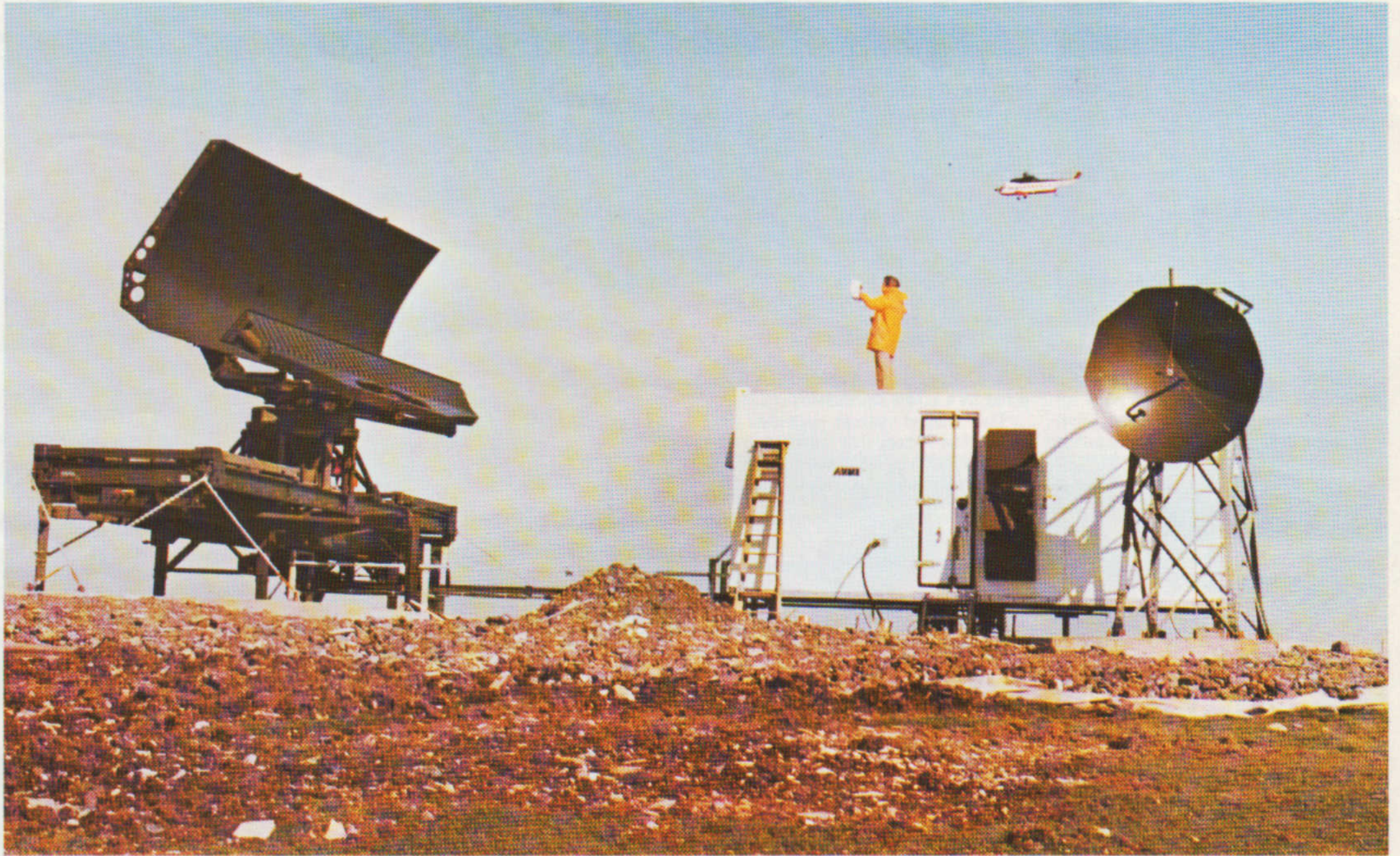
The antenna and S2011 transmitter/receiver undergo on-site tests
