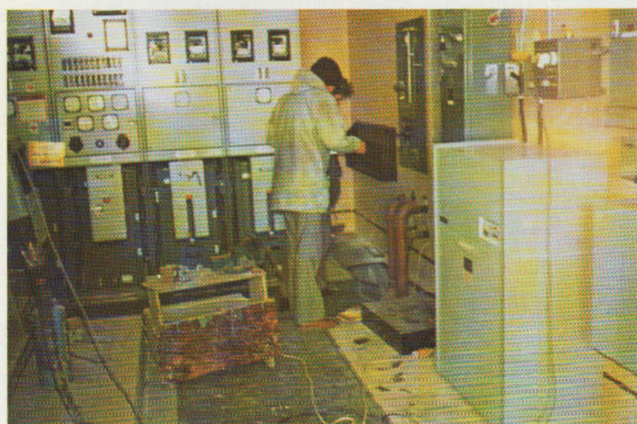
Preparing for an equipment load test
