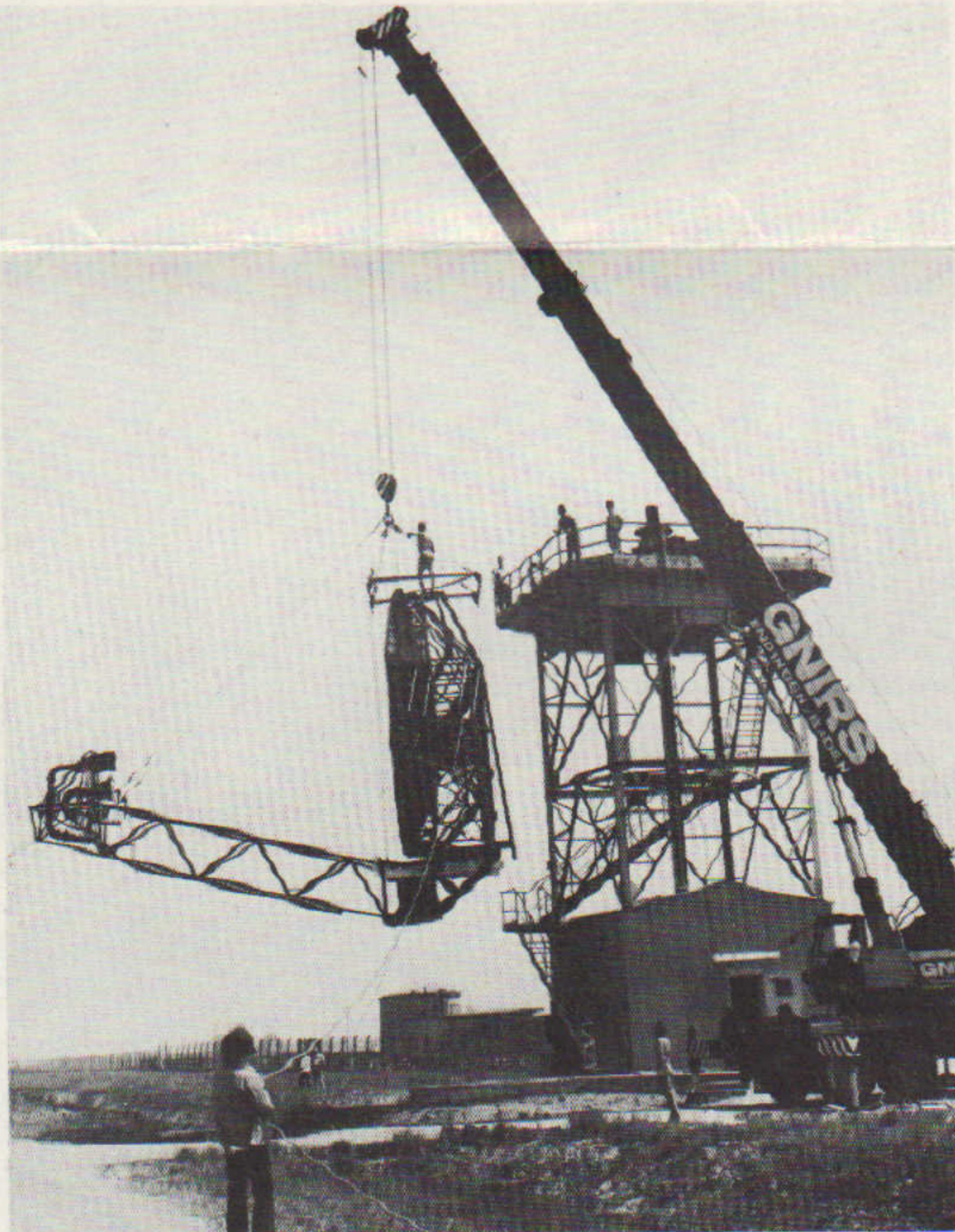
Marconi S654 radar head being installed at Lahr, West Germany
