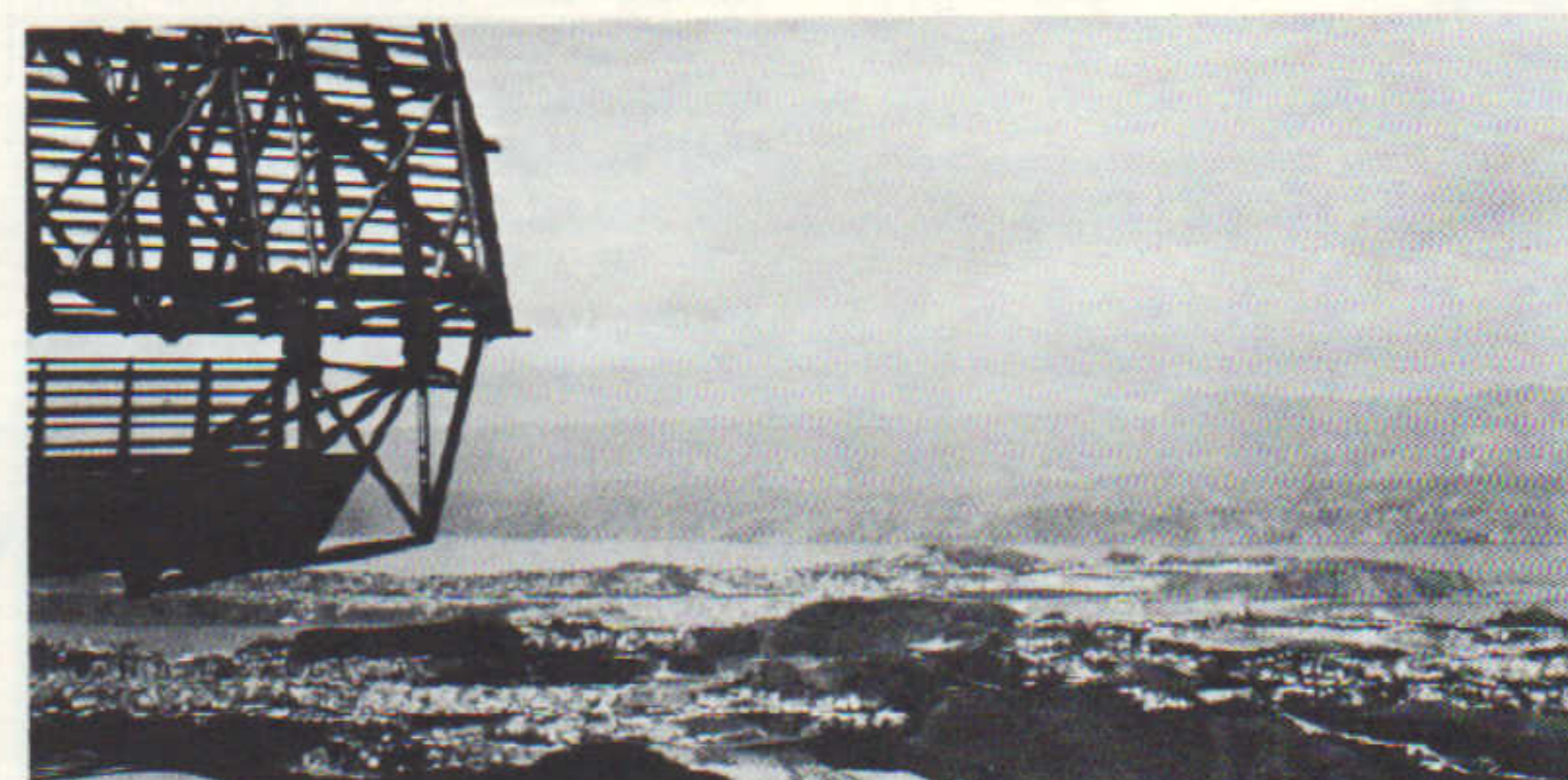
New Zealand: ATC centre at Wellington
