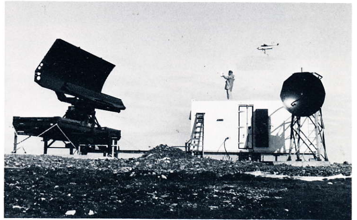
A S1061 radar was installed at Sumburgh Head, the most southerly point of the Shetland Islands, to cope with the rapidly increasing air traffic serving the offshore oil industry. Here the antenna and S2011 transmitter/receiver undergo on-site tests.
