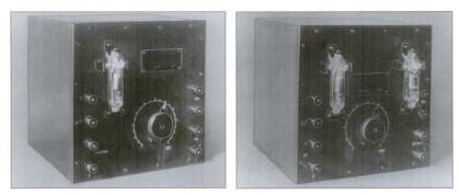
Early prototype detector (left) and amplifier (right) using Marconi patented V24 valves Source: Murray R.P. (2005) "The Early Development of Radio in Canada, 1901-1930"
