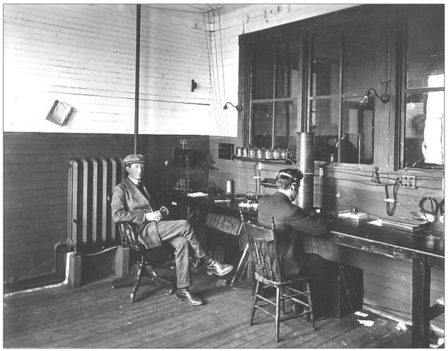
Marconi used Fleming Valve as detectors in the Glace Bay station as early as 1907; a row of 7 spare Fleming valves can be seen lined up to the left of the wireless operator. Marconi is seated on the left Source: Jim Kreuzer, New-York State
