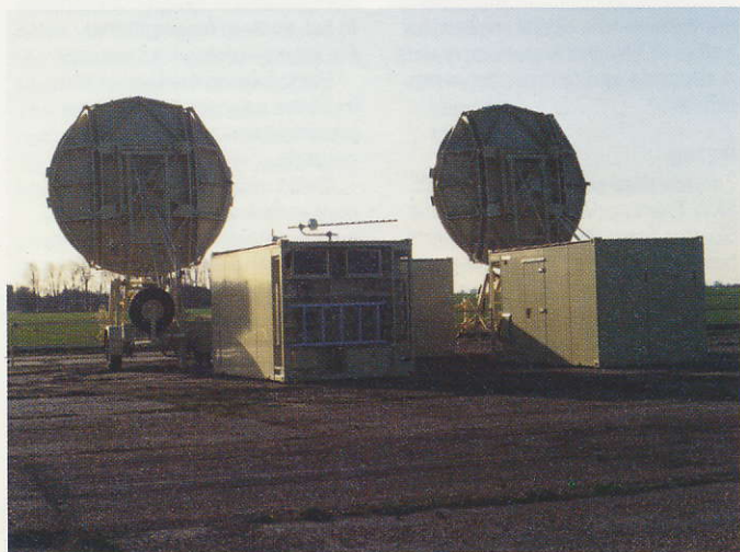
Typical TACTROP/COMCEN terminal complex
