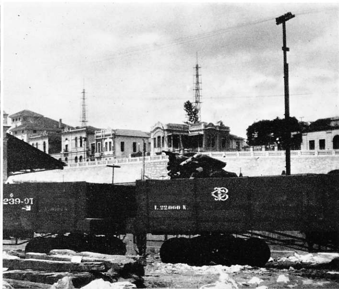
A wireless installation on the Oeste de Minas railway forty years ago. The towers are built of rails.
