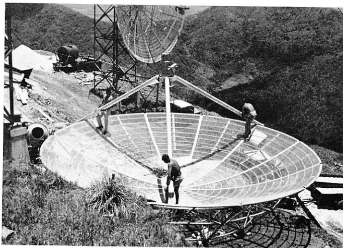
BELOW: Boggy Peak, Antigua—the highest point on the island and chosen for the tropospheric scatter link with St. Lucia, due to go into action this month. With one 30ft. dish towering behind them, Ron Hudson and Bob Hughes, both of Felling M.P.D., work on the aluminium net surface of a second dish. On the roof of the building to the left of the picture can be seen the 4ft. dish for the 7,000 Mc/s link to the Cable and Wireless C.T.O. at Clare Hall, St. John's
