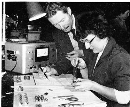
LEFT: Ferrox cube inductances for the AD 308 are made in Coilwinding by Mrs. Joan Broadhead. The Methods engineer who has steered this equipment through from the drawing-board stage to final packing and despatch is Geoff Parry. RIGHT: The main chassis of the AD 308 being wired by Bert Burden. With him here is Ray Dormer, left, Leading Hand
