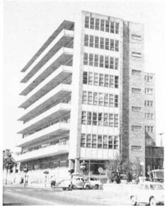
The Page chest pavilion of the Royal Prince Albert Hospital, Sydney. The operating theatre is on the first floor, the studio on the fourth and the lecture hall in the nurses' home, a 1400-foot cable-run away
