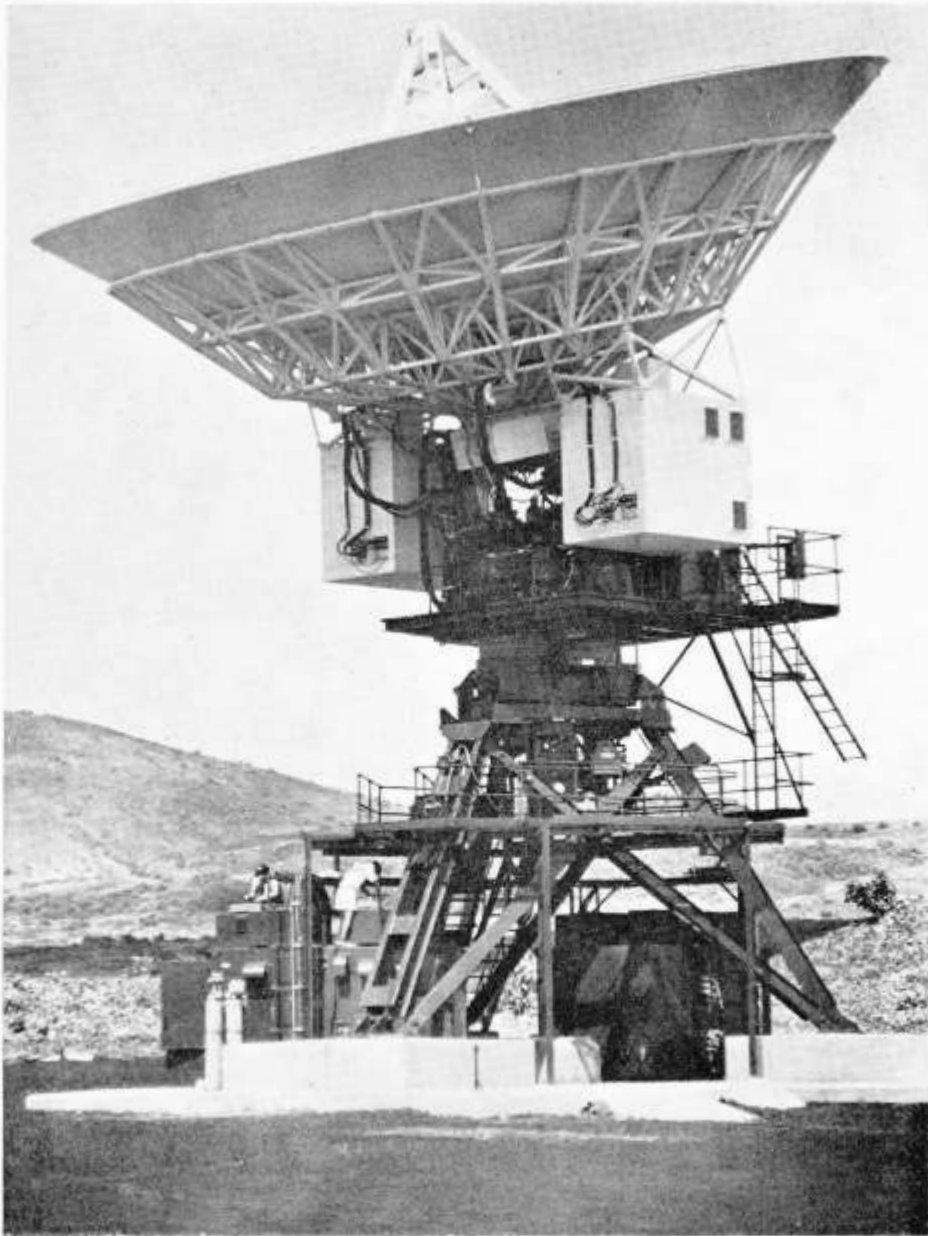
Fig.5. The completed antenna shown in its operational attitude with the transmitter cabins horizontal under the reflector and the power-supply cabins under the gantry legs
