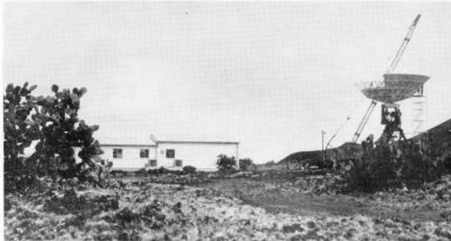
Fig.2. The site during construction with the antenna in course of erection
