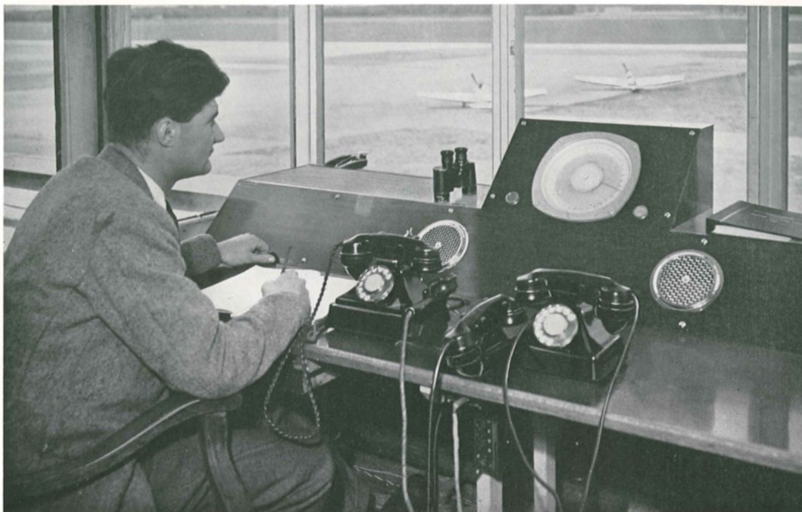
Flying control. ABOVE: a present-day installation showing the remote bearing indicator of the Type AD 200 Direction Finder neatly fitted into the control desk.
