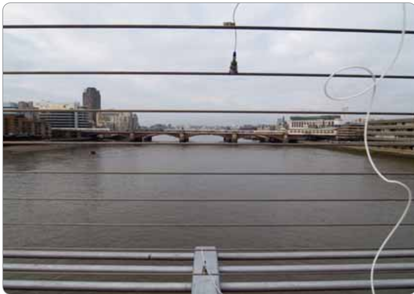
Accelerometers on London's Millennium Bridge track its dynamic vibrations (above) – and replay them as sound in the adjacent Tate Modern gallery (below)
