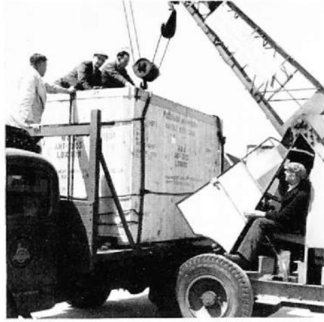
New machinery arriving at the Works is unloaded and installed by mechanical maintenance teams, and wired by the electricians
