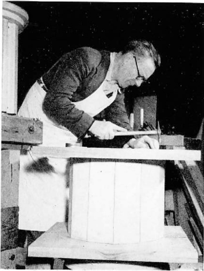
Patterns for metal castings are made of whitewood and mahogany. Fred Joyce is finishing a core box for a sand mould.
