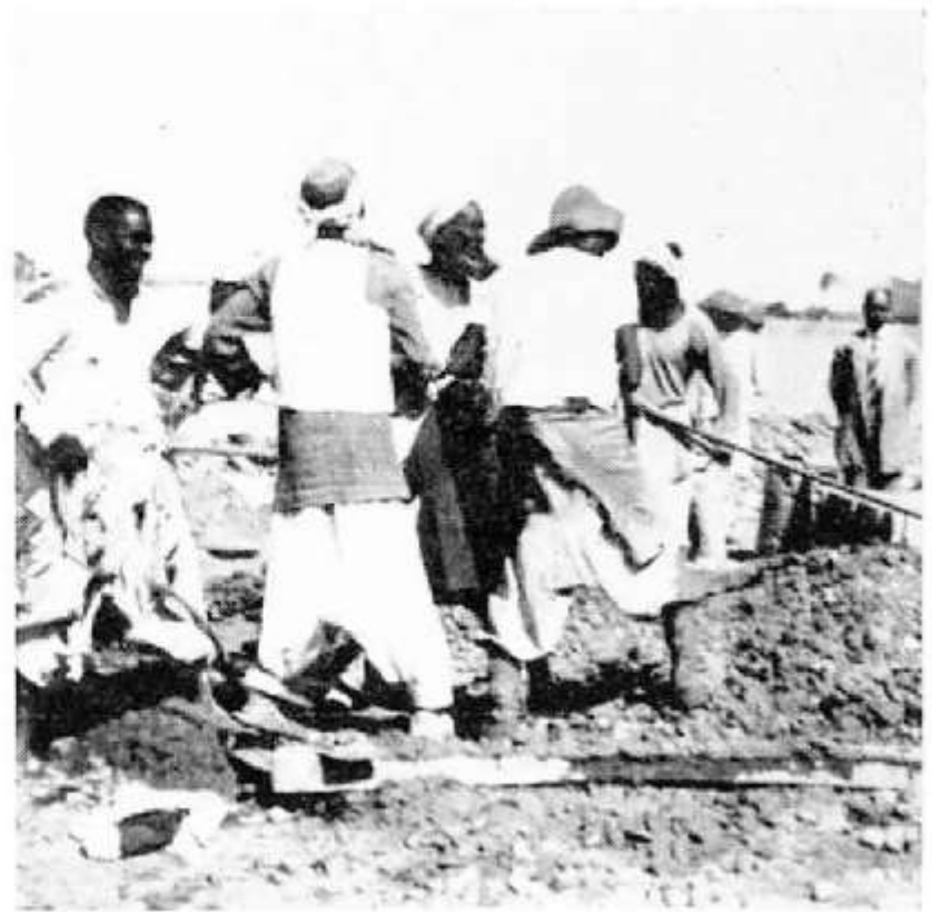
One of the masts erected for the broadcast transmitting station at Abu Zaabel in Egypt. Below, local Arab labourers laying concrete foundations to support the mast stays
